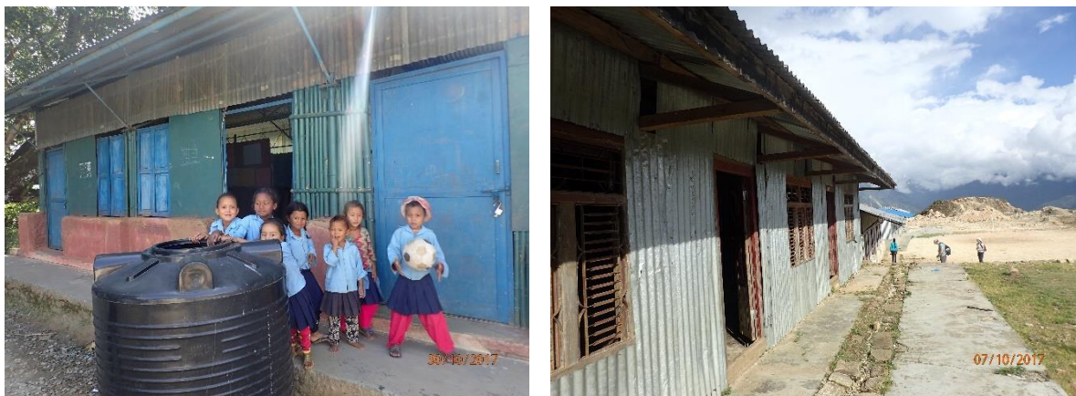
Fig.1 - Examples of Temporary Learning Centre construction, at schools visited during fieldwork, one constructed using bamboo, and one with corrugated sheet metal
