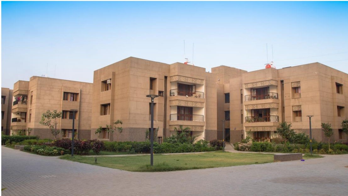
Fig. 5 – Completed CM housing at the IIT Gandhinagar campus, Palaj, Gujarat [33]
