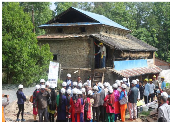
Fig. 7 – Masons receiving hands on training on retrofitting (left) and Representatives from a rural municipality observing the ongoing retrofitting of a typical rural stone masonry building. © NSET
