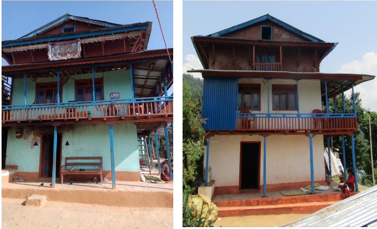
Fig. 8 – A typical 2 storey and attic stone masonry building before and after retrofitting. Beneficiaries are especially attracted to the low levels of architectural interventions thus ensuring adequate usable space.
