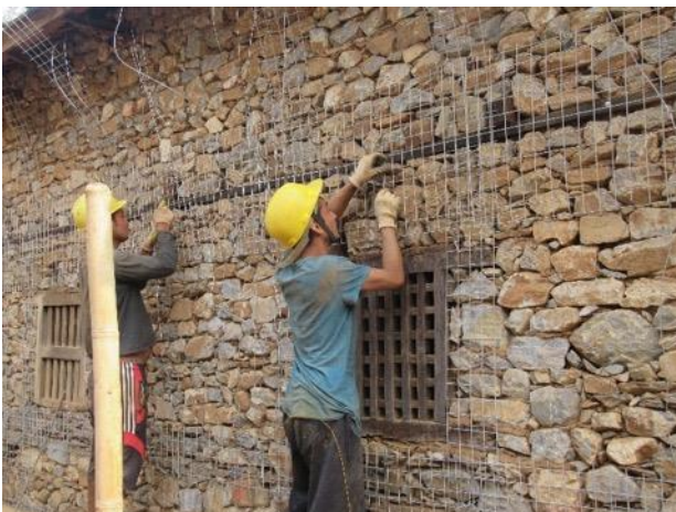
Fig. 7 – Masons receiving hands on training on retrofitting (left) and Representatives from a rural municipality observing the ongoing retrofitting of a typical rural stone masonry building. © NSET
