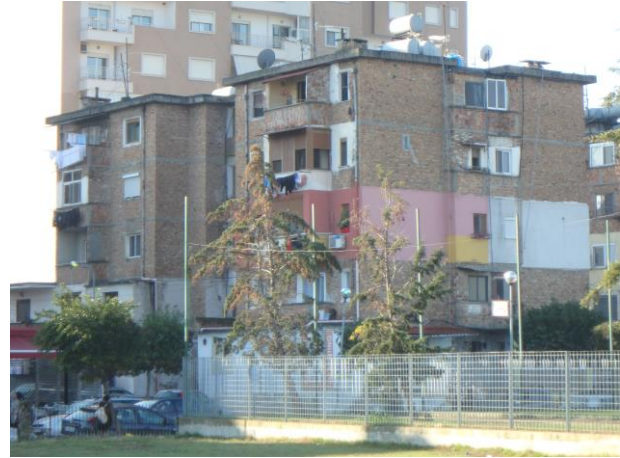
Fig. 3 – Undamaged unreinforced multistory masonry buildings in Durrës, Albania after the Nov. 2019 EQ.
