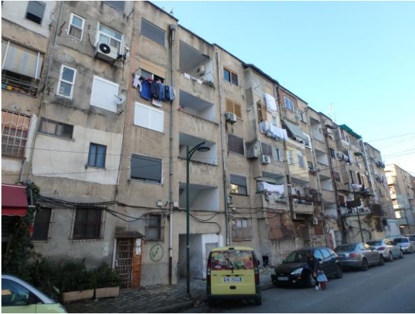
Fig. 3 – Undamaged unreinforced multistory masonry buildings in Durrës, Albania after the Nov. 2019 EQ.
