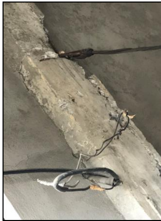
(a) Portion of column removed
