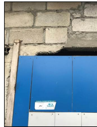
(c) Portion of beam removed
