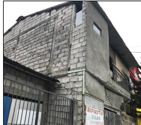
(b) Survey Photo, June 2019
