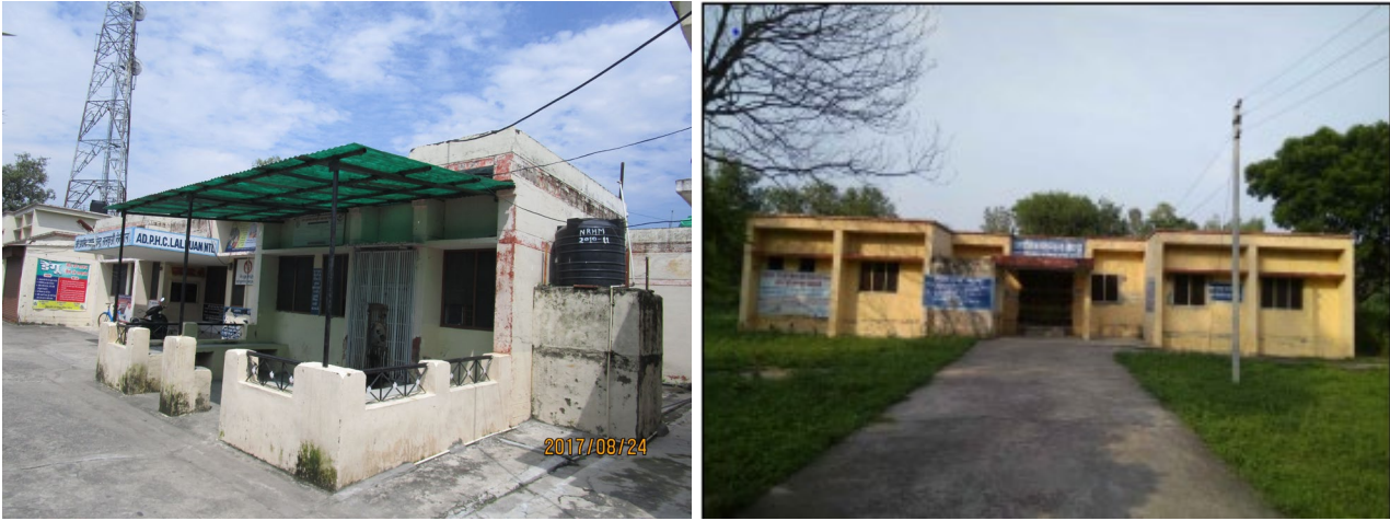
Fig. 2 – Hospital Buildings in Lalkuan, Nainital and Kota Muradnagar, Haridwar
