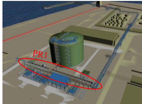
Fig. 1 – Ethylene terminal layout and the RC pipe rack under consideration next to the storage tank
