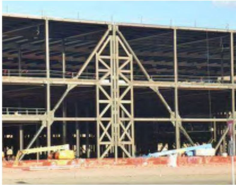
Figure 9 Typical BRB Gueded Fused Strong Back
