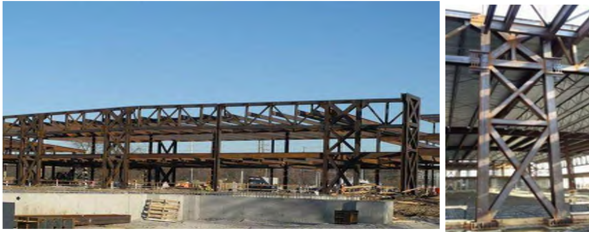
Fig. 7 Construction Photos of the Pre-stressed Fused Rocking Frame System.
