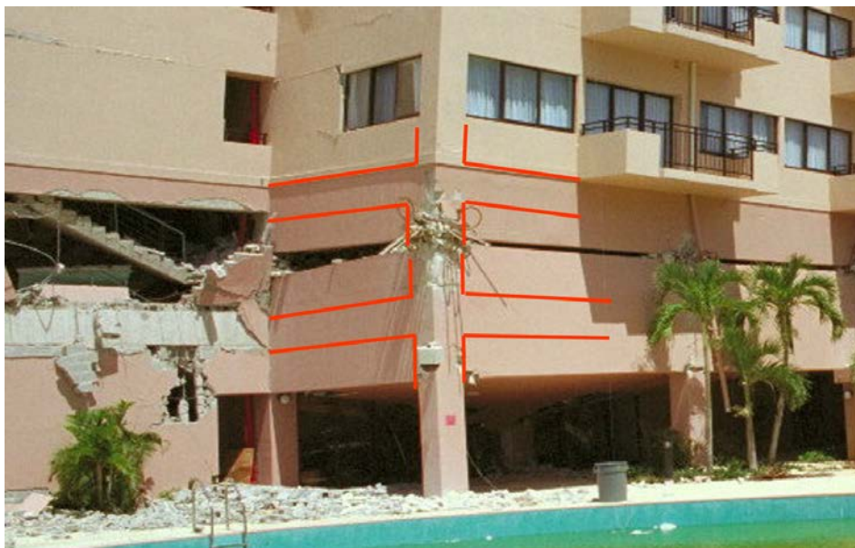
Fig. 2 – Royal Palm Resort – beam, column, and non-structural elements outlined.
