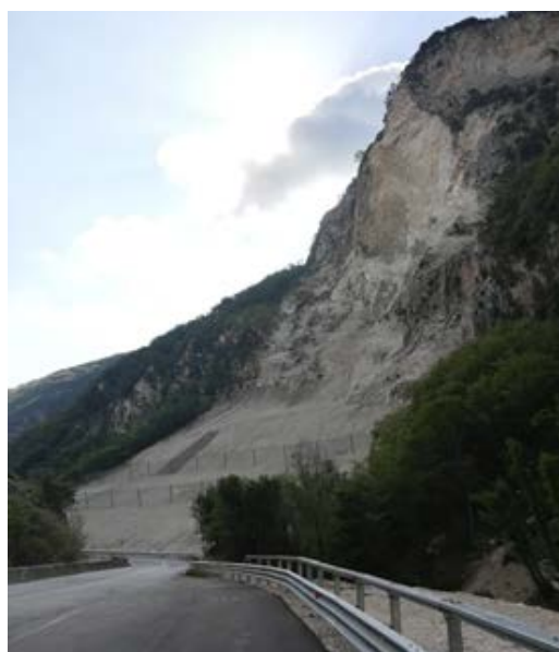
Fig. 5 - The sp 209 near Visso after the interventions (July 2018) [12]
