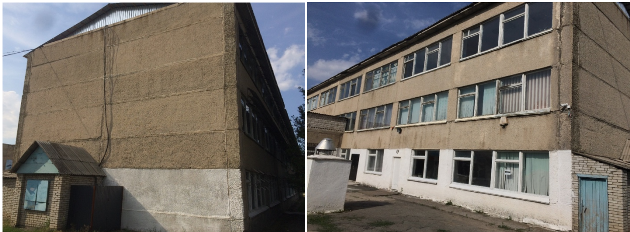
Fig. 4 – Typical PC classroom block in Kyrgyz Republic.
