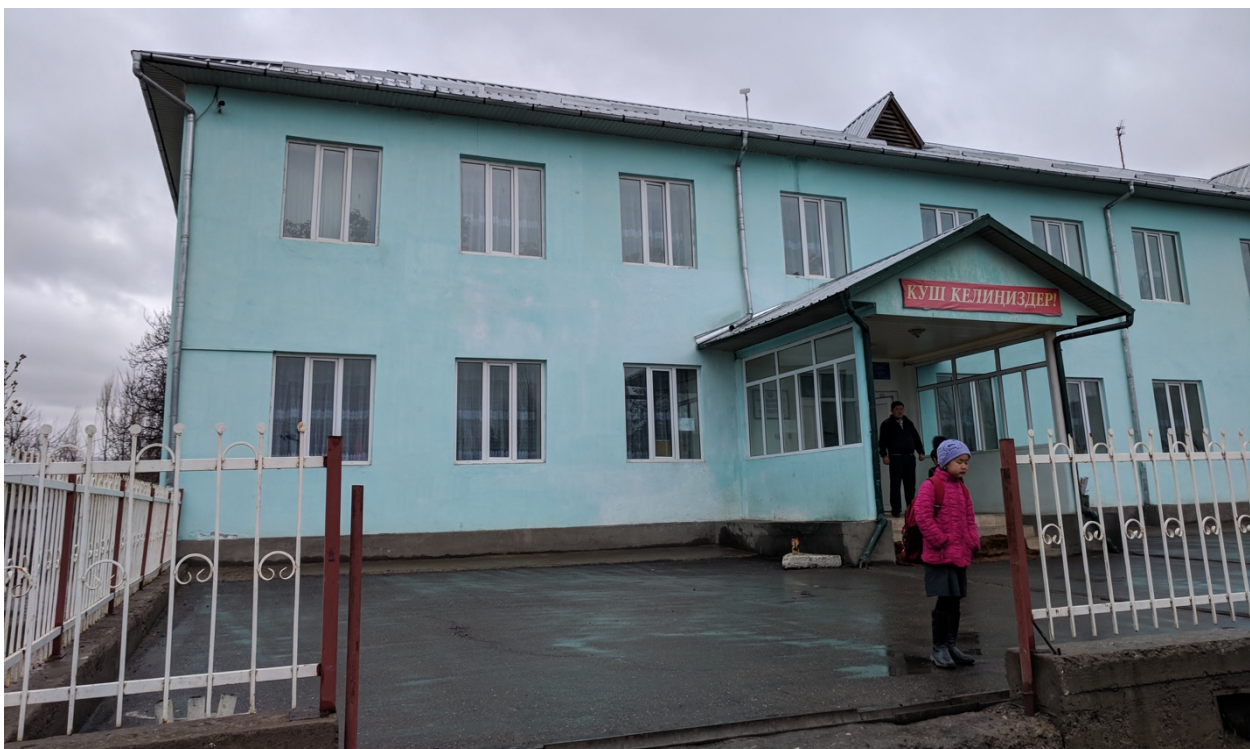
Fig. 2 – Two-story CX school building in Osh.
