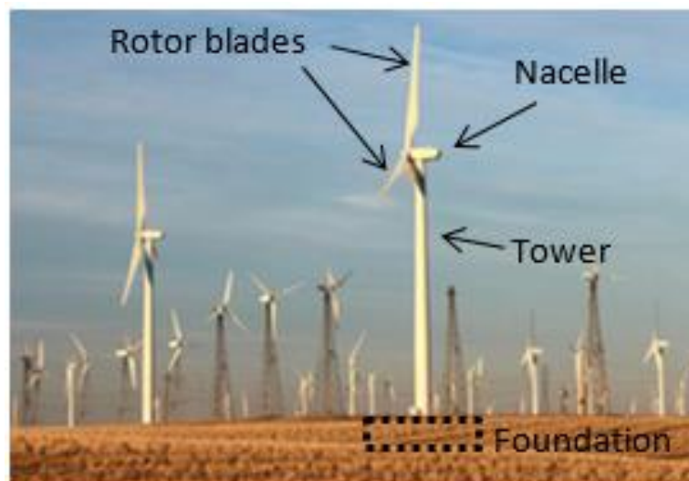
Fig. 4 – Typical wind farm and structure of wind turbines
