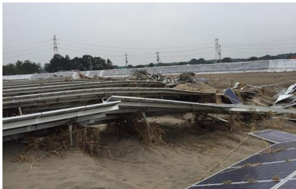
Fig. 13– Example of damage to solar farm (2015 Kanto flood, Japan)
