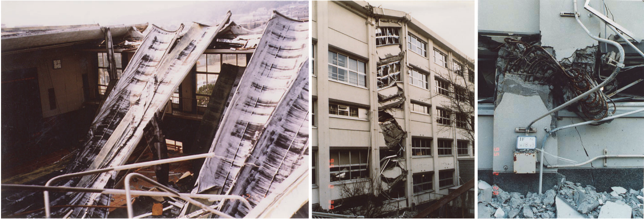
Photo 1: Serious damage to school buildings (1995 Kobe earthquake) [4]
