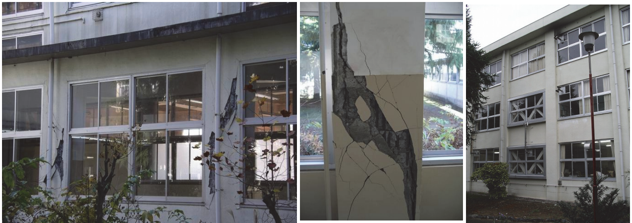
Photo 1: Serious damage to school buildings (1995 Kobe earthquake) [4]
