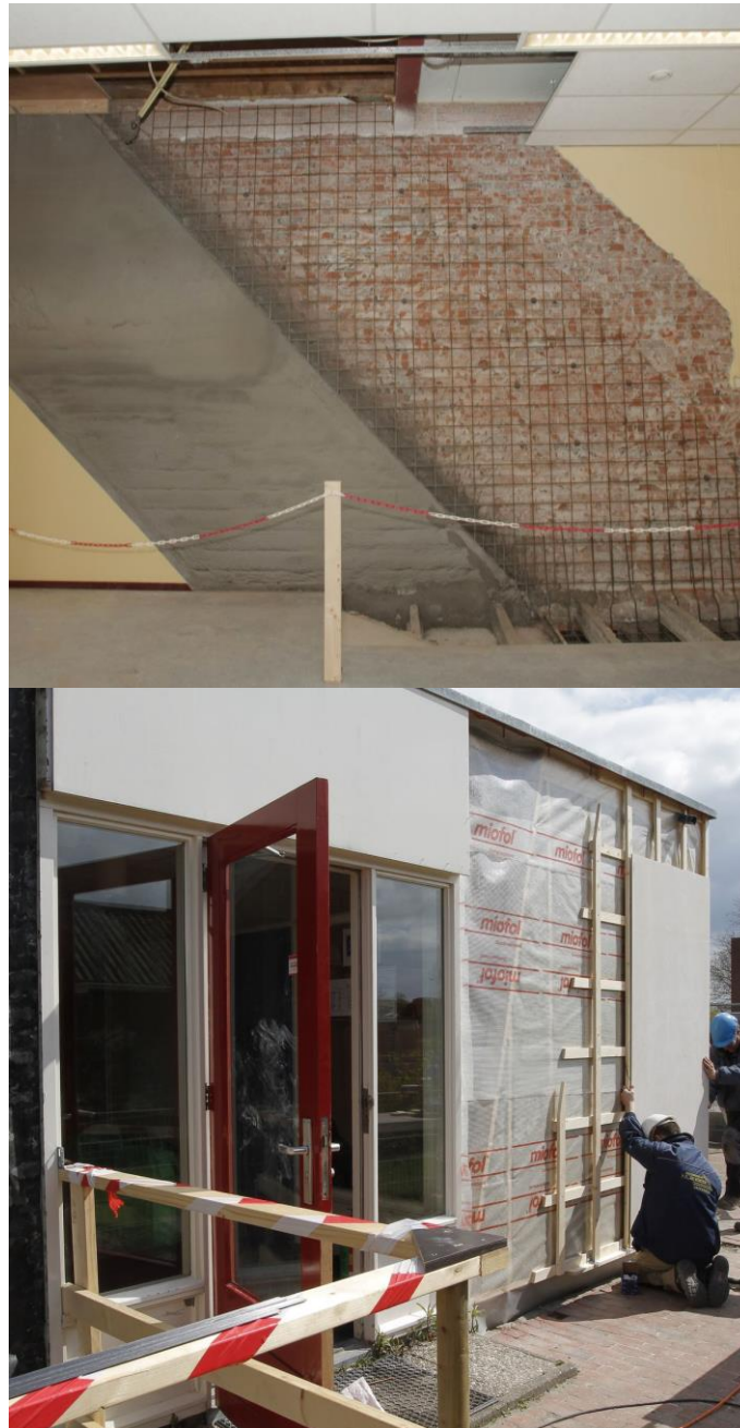
Fig. 9 – Measure L5-A (topside) and L4-J (bottom side) showcased. The measures are built up to show ‘the inside’ of a measure. This in order to explain the impact to the public and to gather feedback from professionals
