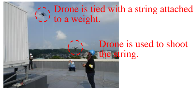
Fig. 8 – Incline angle measurement using a drone
