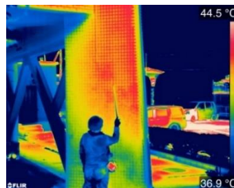
Fig. 10 – Column shot by the infrared thermography camera
