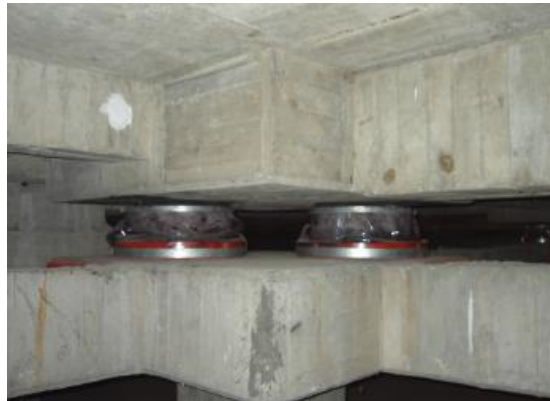
Figure 5 Ball isolator devices
