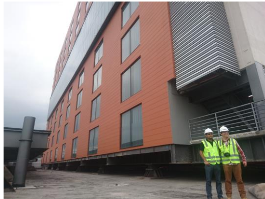
Figure 3 Isolator Building Hotel Via Vallejo
