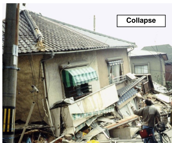
Photo 1: An example of ordinary “severely damaged” buildings and “collapsed” buildings
