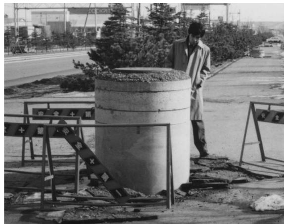
**Figure 4: Uplifted manhole in Kushiro-cho (Courtesy of Mr. Y. Suzuki)**
