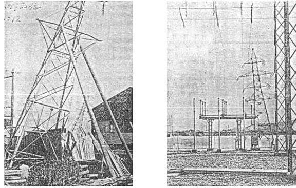
**Figure 1: Inclined power transmission towers seen after Niigata earthquake, 1964**
