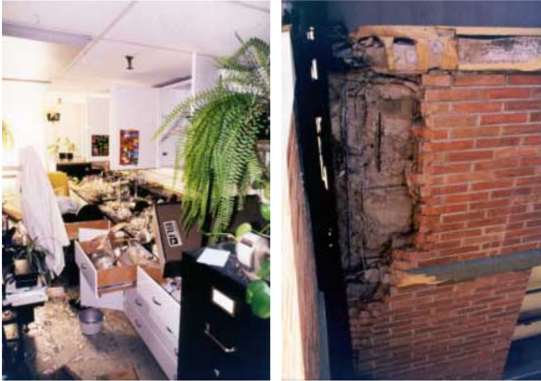
Figure 1: Left photo shows typical earthquake damage to contents in laboratory space.
