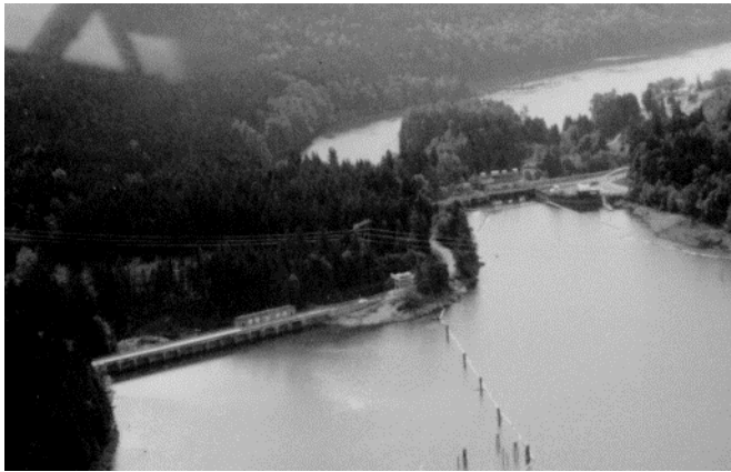
Photo No. 1 Blind Slough Dam (on left) and Stave Falls Main and Intake Dams
