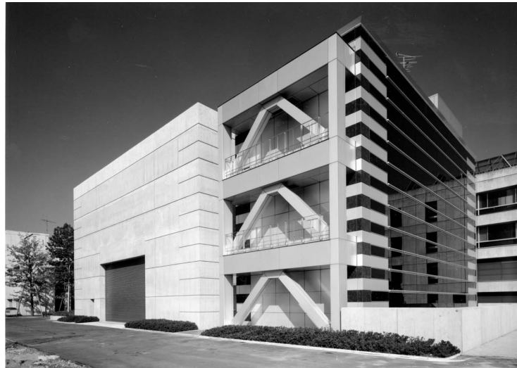
Fig.1 3-Story building with Active Variable Stiffness system
