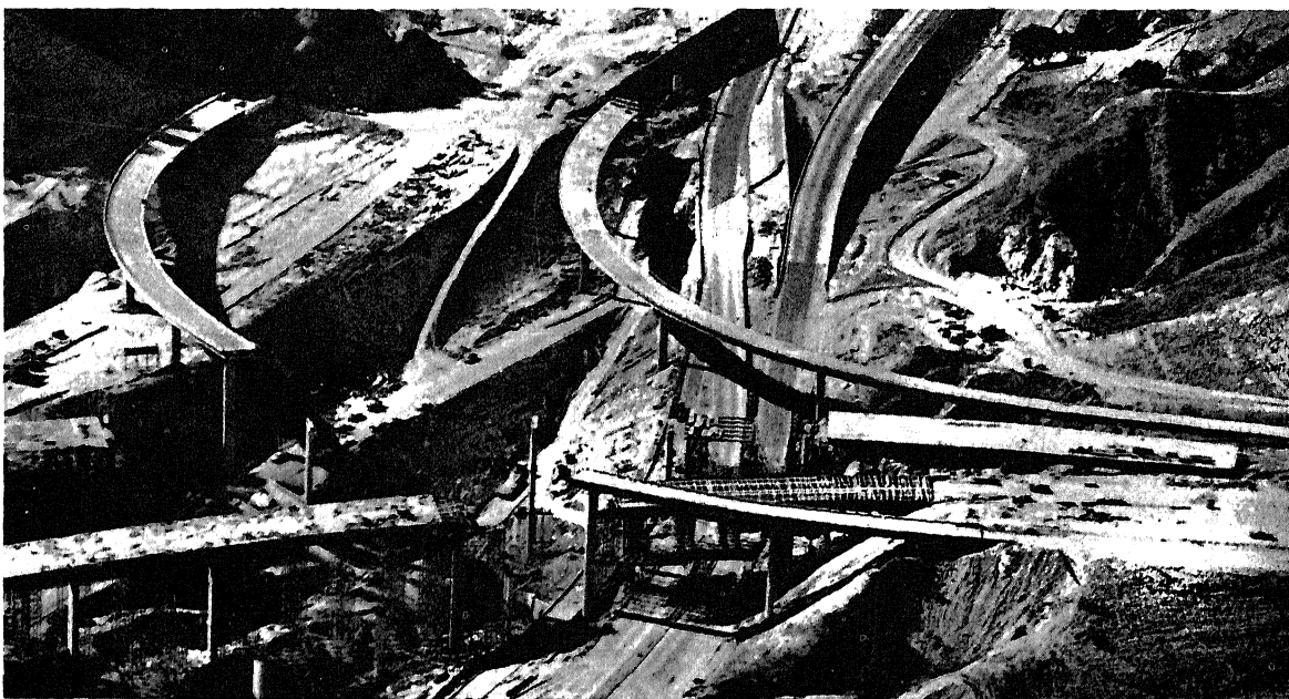
Figure 2 Post-earthquake view, looking west, of the Golden State-Antelope Valley freeway interchange. The center two spans of the highest overpass have collapsed. Photographed by Ralph Samuels
