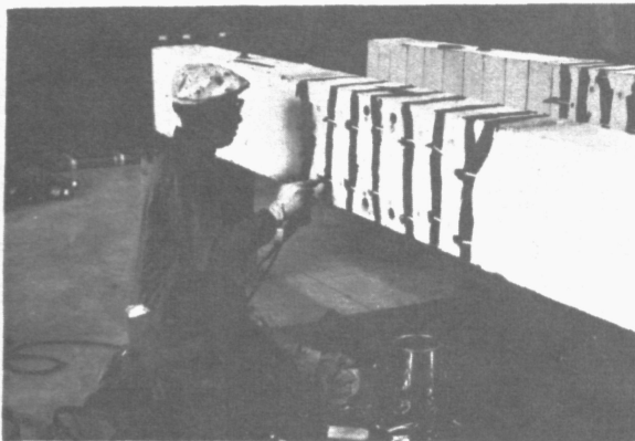
PHOTO 3 REPAIR OF BEAM
