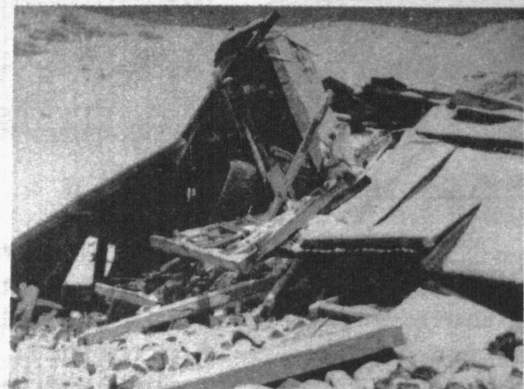
FIG.7 - COMPLETE COLLAPSE OF A BUILDING IN RRSM IN MUD MORTAR AT LEO
