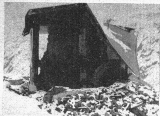
FIG. 4 - DAMAGE TO A DOUBLE STOREY ROADSIDE HOUSE NEAR SHALKAR. IMPACT OF LARGE BOULDER ALSO CAUSED SEVERE DAMAGE.
