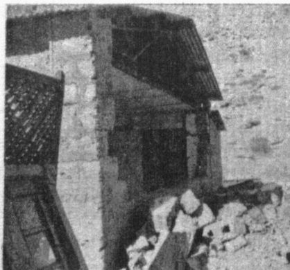
FIG.8 - COLLAPSE OF GABLE END WALL MADE OF HOLLOW CONCRETE BLOCKS NEAR SUMDOH
