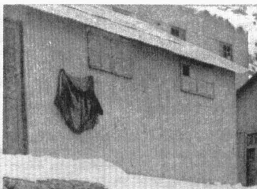
FIG.10 - UNDAMAGED HOUSE MADE OF CORRUGATED IRON SHEETS NAILED ON TIMBER FRAME WITH SLOPING ROOF
