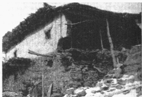
FIG. 2 - COMPLETE COLLAPSE OF SUNDRIED MUD BRICK WALL OF A DOUBLE STOREYED HOUSE AT SHALKAR. THE GROUND FLOOR IS IN RSM IN MUD MORTAR
