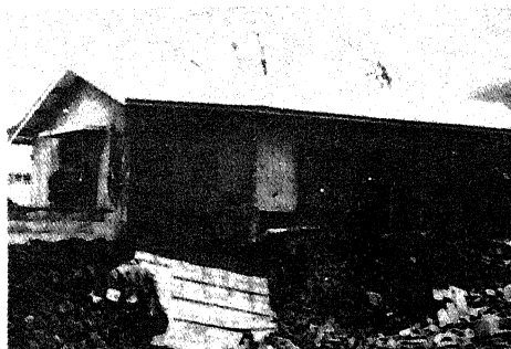
Photo 6. Damage of wooden house with reinforced concrete block wall (Iruma)
