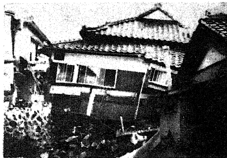
Photo 4. Destroyed house caused by collapse of retaining wall (Iruma)
