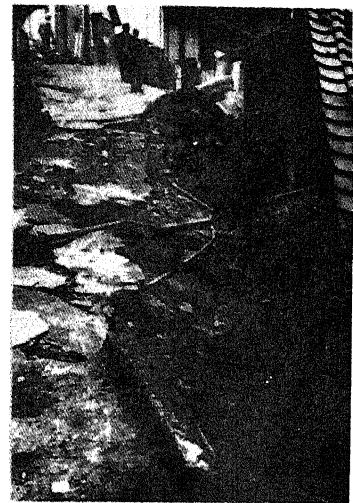
Photo 1. Crack in the ground caused by collapse of retaining wall (Iruma)
