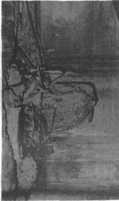
Fig. 10 - Damage to the first story interior long-column at coordinates D-11. Bottom of the column punched through the first-story slab.
