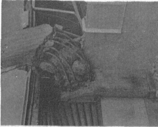
Fig. 10 - Damage to the first story interior long-column at coordinates D-11. Bottom of the column punched through the first-story slab.
