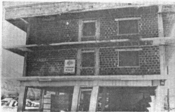
Fig.3 Yielding of first floor columns
