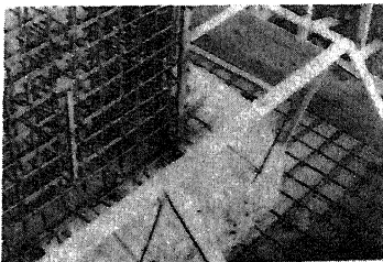
Photo 12. The steel mesh shown was welded to the existing bars. The footing high was increased
