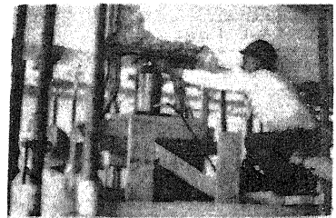
Photo 11. Lifting a settled column
