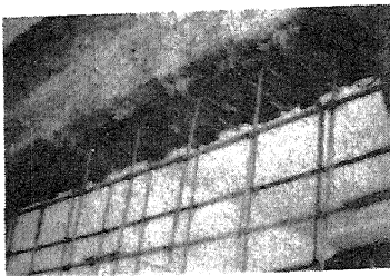
Photo 10. Welding the new shear wall bars to the beam bars
