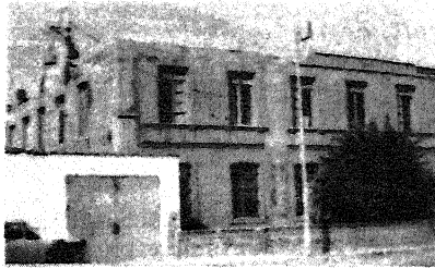
Photo 1. Brick building. Note that from the post to the left has been reinforced
