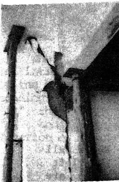
Photo 5. Joint damage
