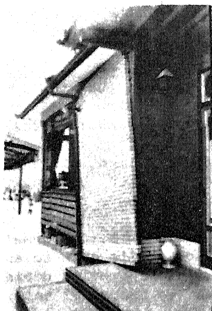
Photo.8. A tiled wall slipped out due to the poor connection to the sheathing.....
