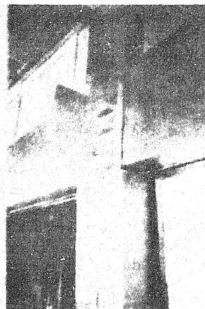
Photo.6. Zig-zag crack at the notch of the column
