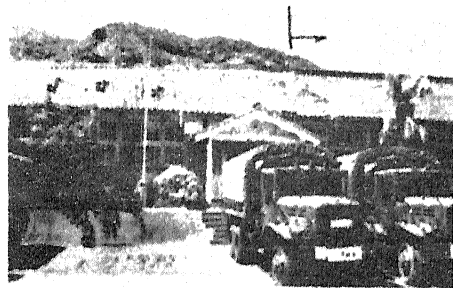
Photo.4 Remarkable difference of the damage of roof tiles is caused by the rigidity of the roof structure.
