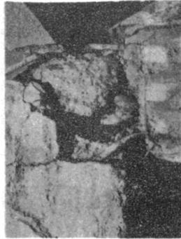
(d) Case K. Inadequate anchorage of beam reinforcement in exterior frame joint, together with no confinement of joint
