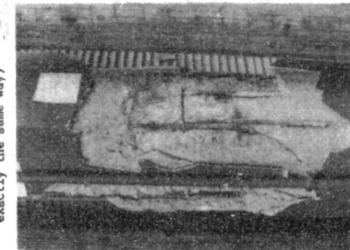
(c) Case J. Poor reinforcement joint. Lack of stirrups, small concrete cover and inadequate overlapping
