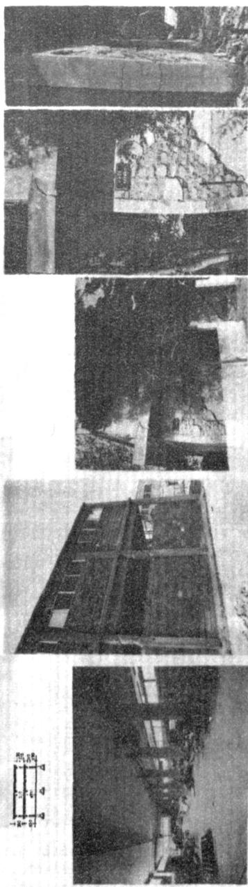
(e) Case B. Two storey factory building. Free interior column. Perimetrical columns act with a short free height, due to masonry infill. Compare also with fig. 2.5A
