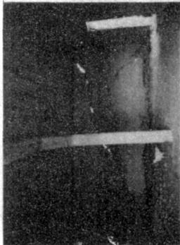
(a) Central column with plastic hinges at ends. Riffs are 40 cm. Median quality of construction. Not designed for EQ.
