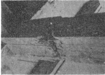
(b) Case I. Poor construction joint, not reinforced properly (12 columns of the same building were damaged in exactly the same way)
