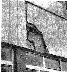
Fig.5-Damage at expansion joint
