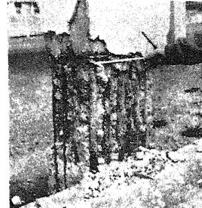
Fig.7-Detail of column hinging
