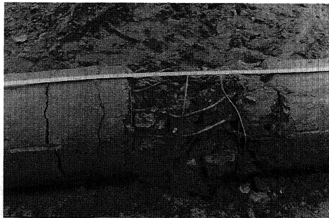
Photo 2 Damage of a Pile
