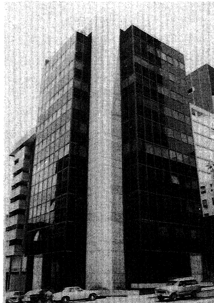
Fig. 9 - Building with corner Box-shaped Shearwalls.
