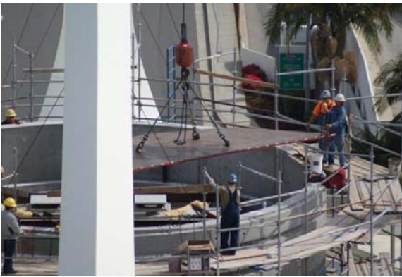
Figure 29. Steel plate placement
