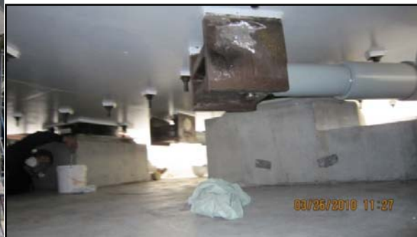
Figure 30. Bearings and dampers
