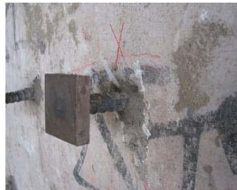
Figure 18. Lap splice retrofit
