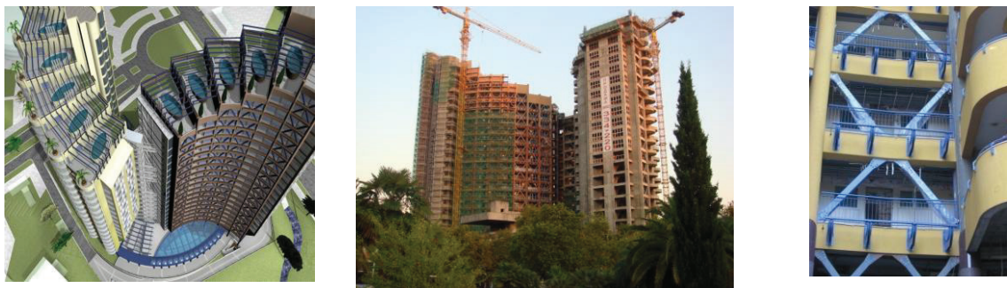
Figure 7. Apartment housing estates «New Alexandria» with damping system of metal braces
