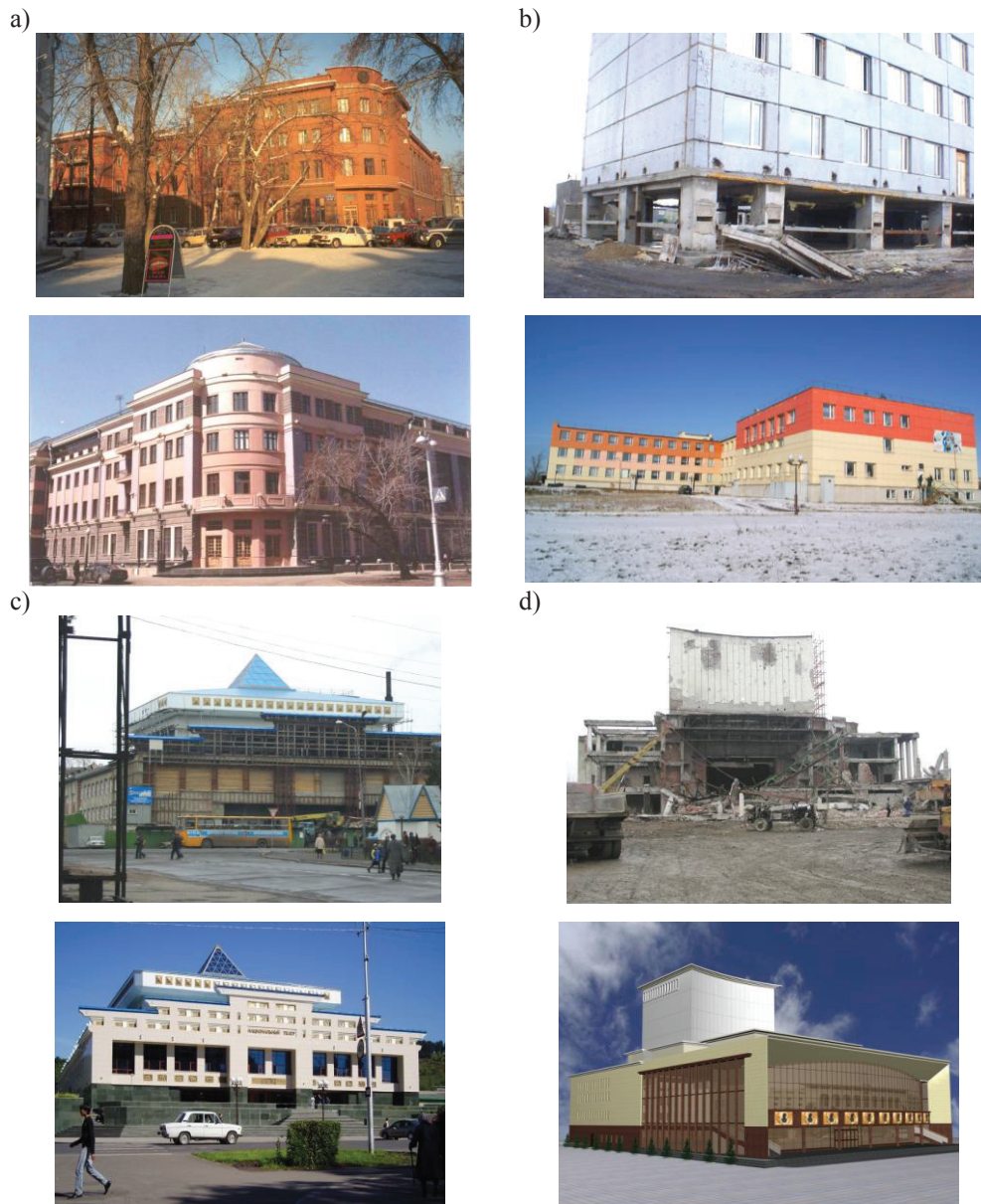
Figure 3. Use of seismoisolation supports to provide buildings seismic resistance a) the reconstruction of historical building of bank in Irkutsk; b) four buildings of school in Aleksandrovsk-Sakhalinsky; c) seismic strengthening of theater building in Gorno-Altaysk; d) reconstruction of the building of concert hall in Grozny, destroyed by military operations
