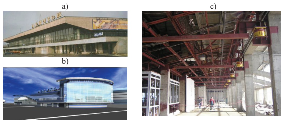
Figure 8. New solution for seismic protection of the building of Irkutsk Civil Airport a) airport building before reconstruction; b) airport building after strengthening; c) the energy dissipation elements in working condition
