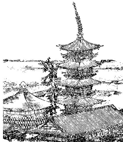
Fig.1 Damage of decorative pole of five-storeyed pagoda in Tokyo by Great Ansei-Edo Earthquake of 1854 (after F. Ohmori, 1921)
