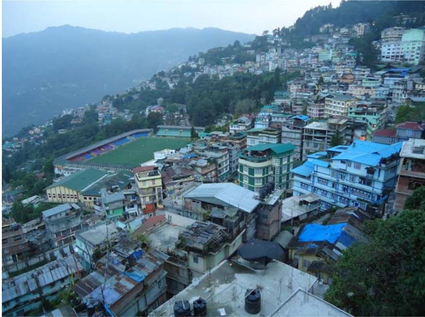
**Figure 1.1** Skyline of Gangtok city covered with RC frame buildings in hill slopes built in last 10-15 years with no techno-legal regime in place
