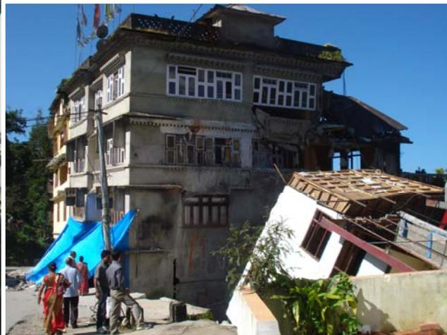
**Figure 2.4** Buildings on slope collapsed during 2011 Sikkim Earthquake: (a) Collapse of intermediate storeys of Dzongpo House in Gangtok, and (b) Adjoining 3-storey building also collapsed
