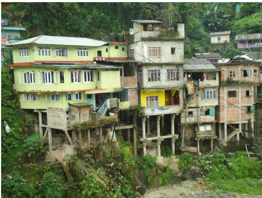
**Figure 1.2** Housing sprawl along the Teesta river side made of reinforced concrete frames, that lack many desirable features necessary to be called earthquake resistant
