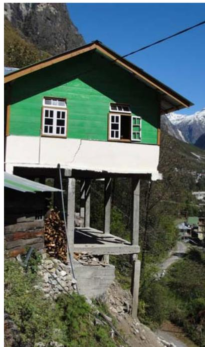
**Figure 2.2** RC frame supports of RC frame buildings on hill slopes are not designed with the basic effects to withstand even small as was noted during the 18September 2011 earthquake
