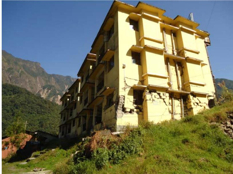
**Figure 2.1** Building by government on shallow slope constructed near Chungthang, North Sikkim, was severely shaking in the first storey during 2011 Sikkim Earthquake. RC corner column is well confined and severely distorted
