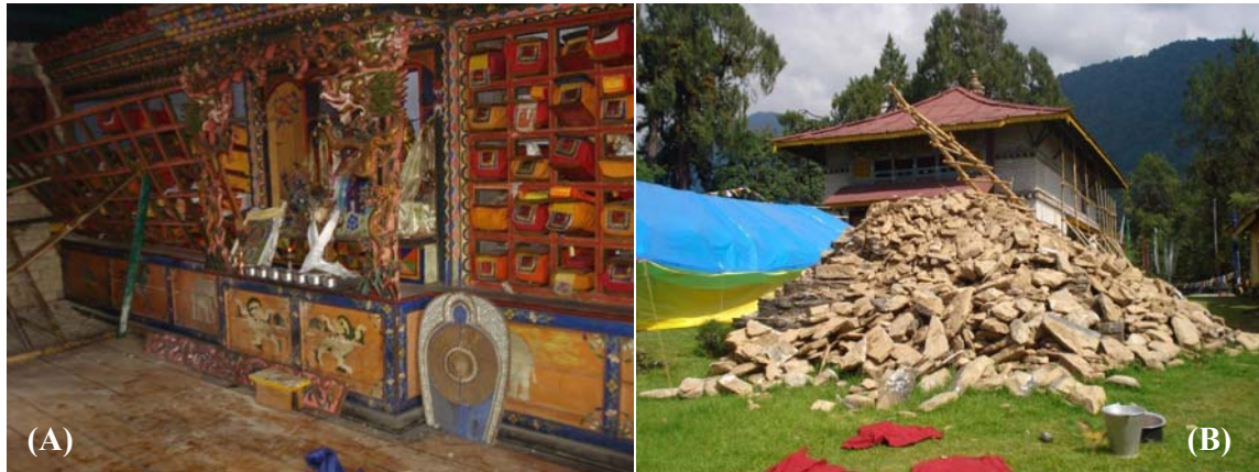
Figure 5. (A) Holy scriptures dislodged from the cabinet in the Dubdi Monastery, Yuksom (B) Collapse of stone masonry stupa in the Dubdi Monastery, Yuksom
