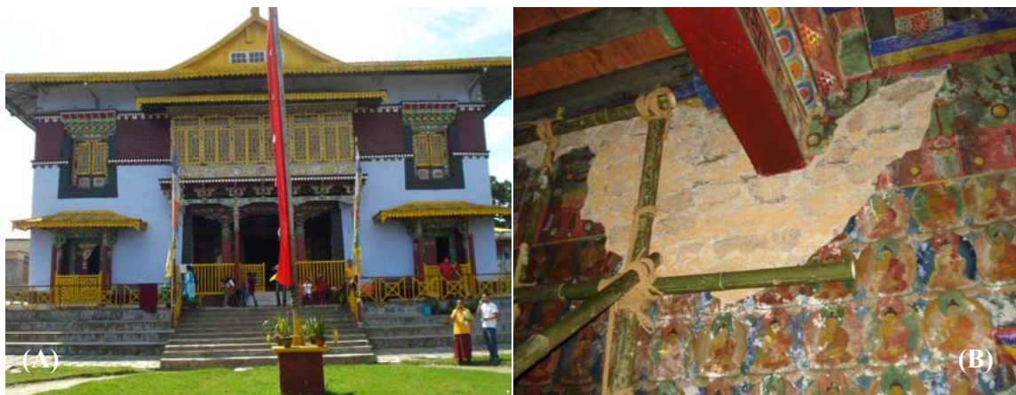
Figure 10. (A) Semi-dressed stone masonry walls with wood frame, Pemayangtse Royal Monastery, Pelling (1705 AD) (B) Out-of-plane damage to stone walls by timber beams resting on them, Pemayangtse Royal Monastery, Pelling
