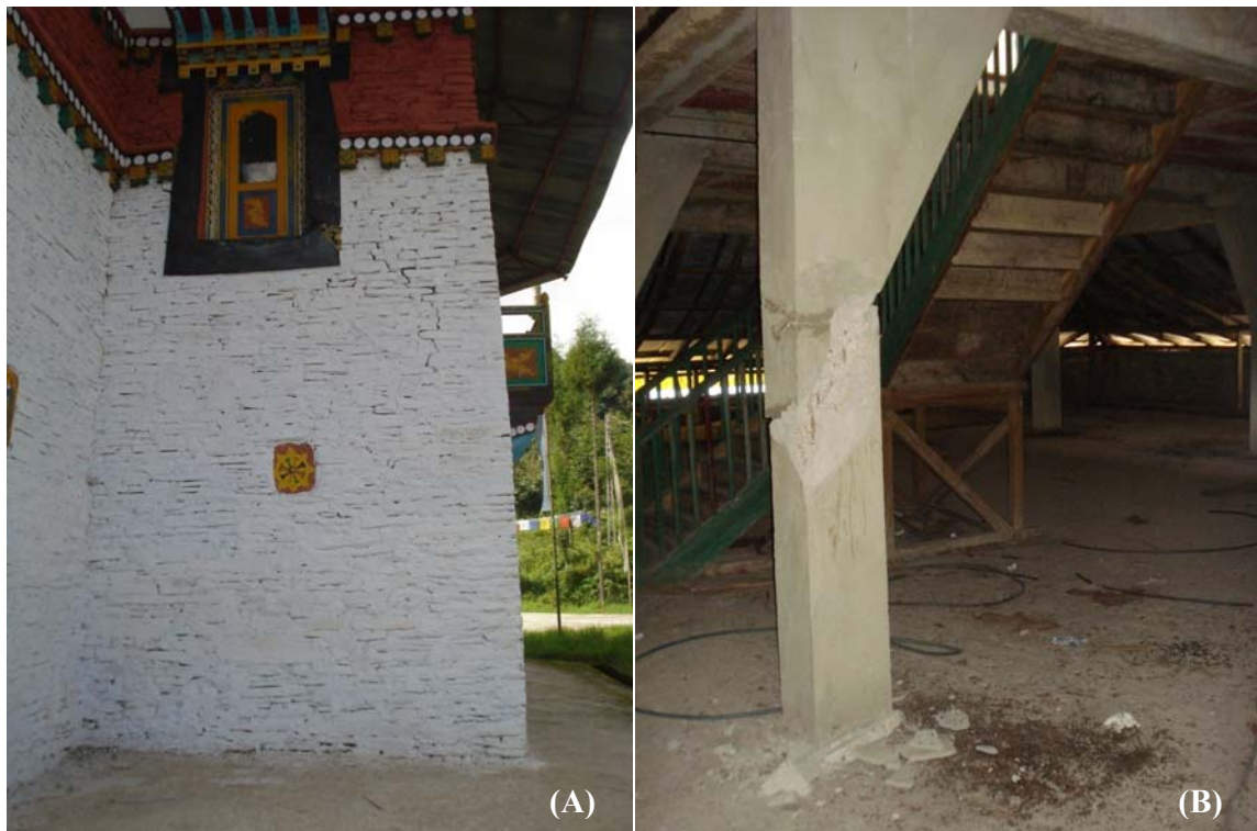
Figure 8. (A) Out-of-plane mechanism in the RR masonry walls in Phodong Monastery, Phodong, (B) Shear failure of RC columns at roof level in Phodong Monastery, Phodong
