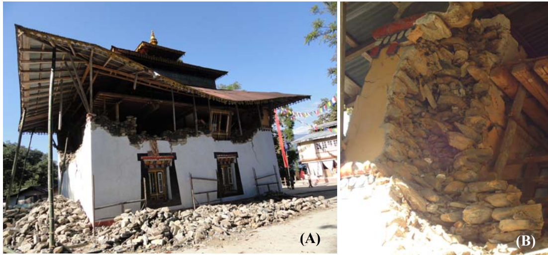
Figure 3. (A) Extensive damage to the RRM structure of the Ringin Monastery in Mangan, (B) Out-of-plane failure of RRM walls of the Ringin Monastery in Mangan
