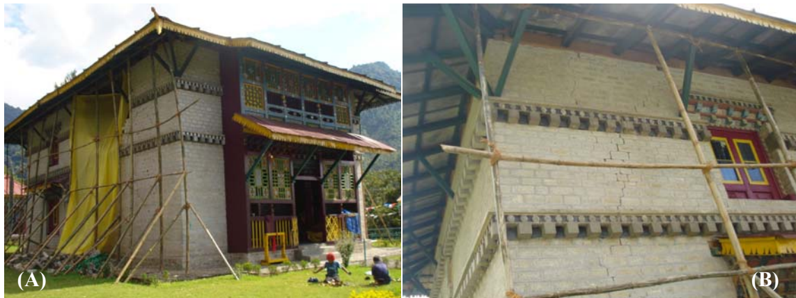
Figure 4. (A) Wood frame structure with semi-dressed stone walls in the Dubdi Monastery, Yuksom, (B) Initiation of out-of-plane mechanism in the semi-dressed stone masonry walls
