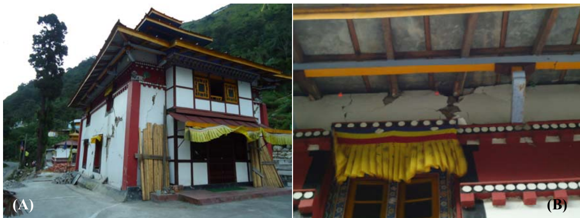
Figure 6. (A) Wood frame with plastered stone masonry walls and RC columns in Chungthang Monastery, Chungthang, (B) Damage to walls from pounding of rafters
