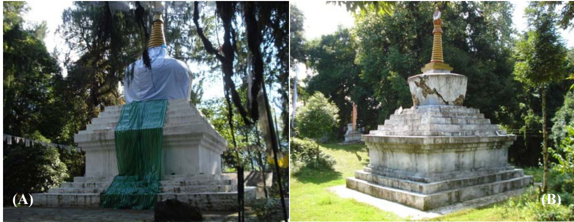
Figure 9. (A) Damaged stone masonry stupa at the Coronation Throne, Norbugang (B) Damaged stone masonry stupa in the Pemayangtse monastery premises, Pelling
