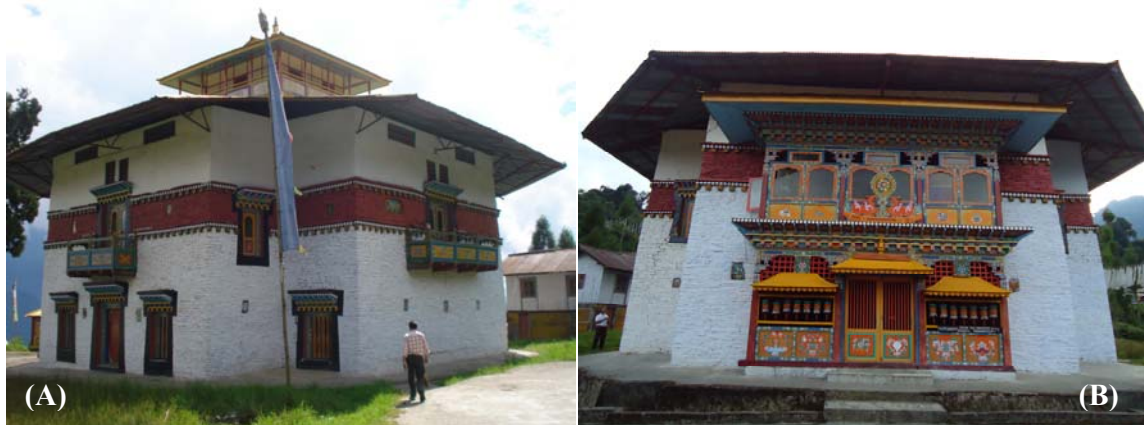
Figure 7. (A) Wood frame with RR masonry walls in Phodong Monastery, Phodong, (B) Wood frame with RR masonry walls in Phodong Monastery, Phodong
