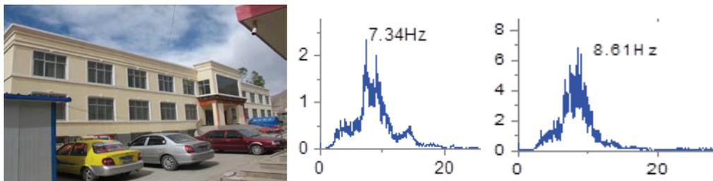
Figure 8. A 2-story CBCM residential building without damage and its' NF (7.34Hz/8.61Hz) tested
