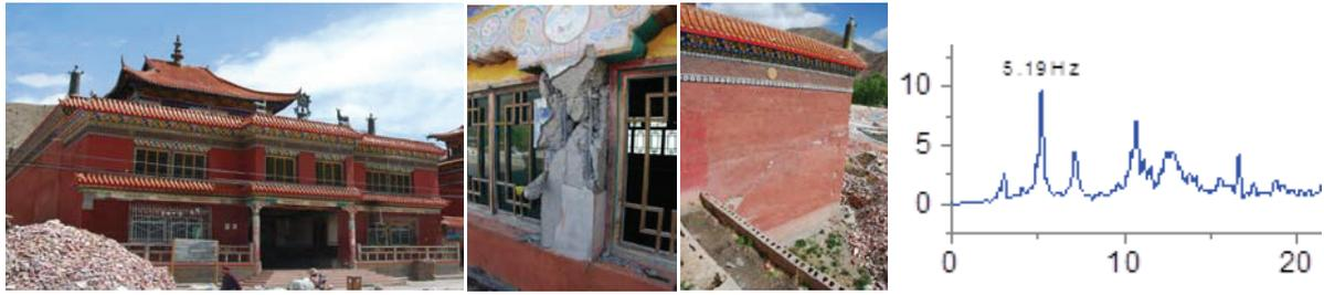
Figure 15. Damage of a 3-story IRCFSMW temple building and its' NF (5.19Hz/5.81Hz) tested
