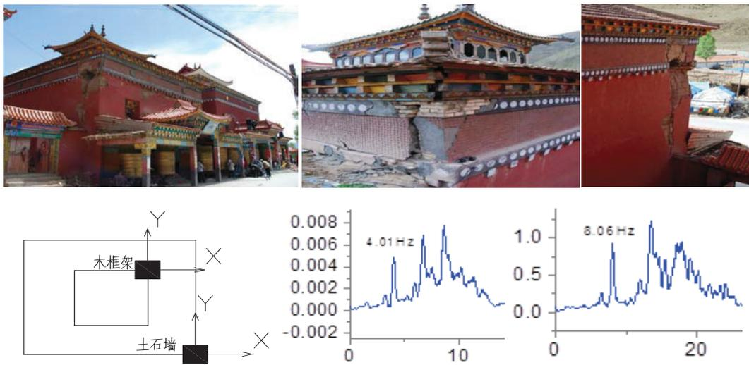
Figure 16. Damage of a 3-story IWFSMW temple building and its' NF (4.01Hz/8.06Hz) tested
