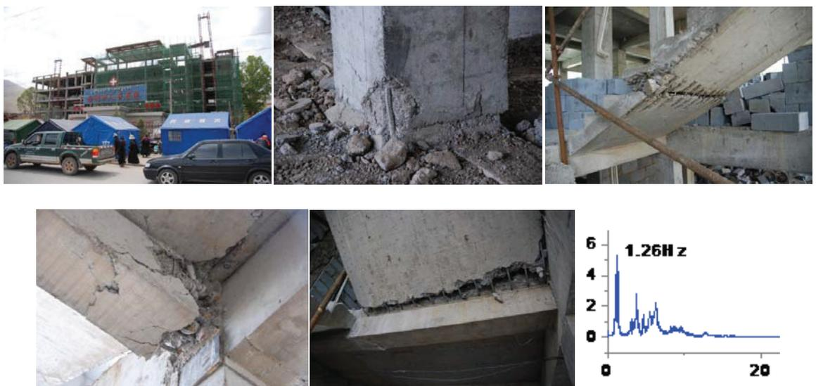
Figure 13. Damage of a 5-story RCF hospital building and its' NF (1.26Hz) tested
