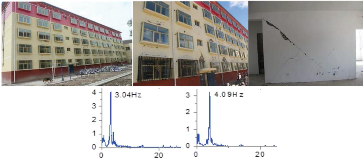
Figure 7. Typical damage of a 5-story CBCM residential building and its' NF (3.04Hz/4.09Hz ) tested
