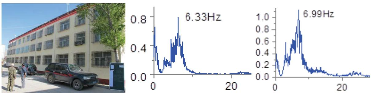
Figure 5. A 3-story LCBCM residential building without any damage and its' NF (6.33Hz) tested
