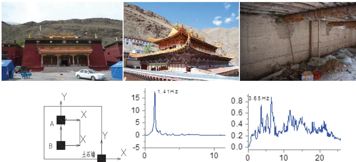
Figure 17. Damage of a 3-story IWFSMW temple building and its' NF (1.41Hz/3.65Hz) tested
