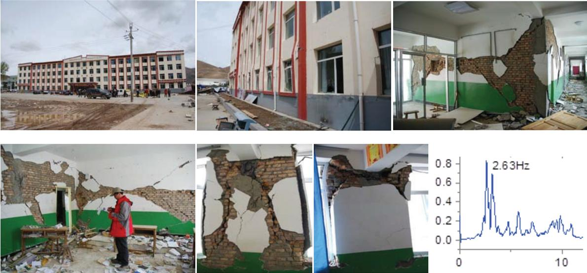
Figure 6. Typical damage of a 4-story CBCM school building and its' NF (2.63Hz) tested
