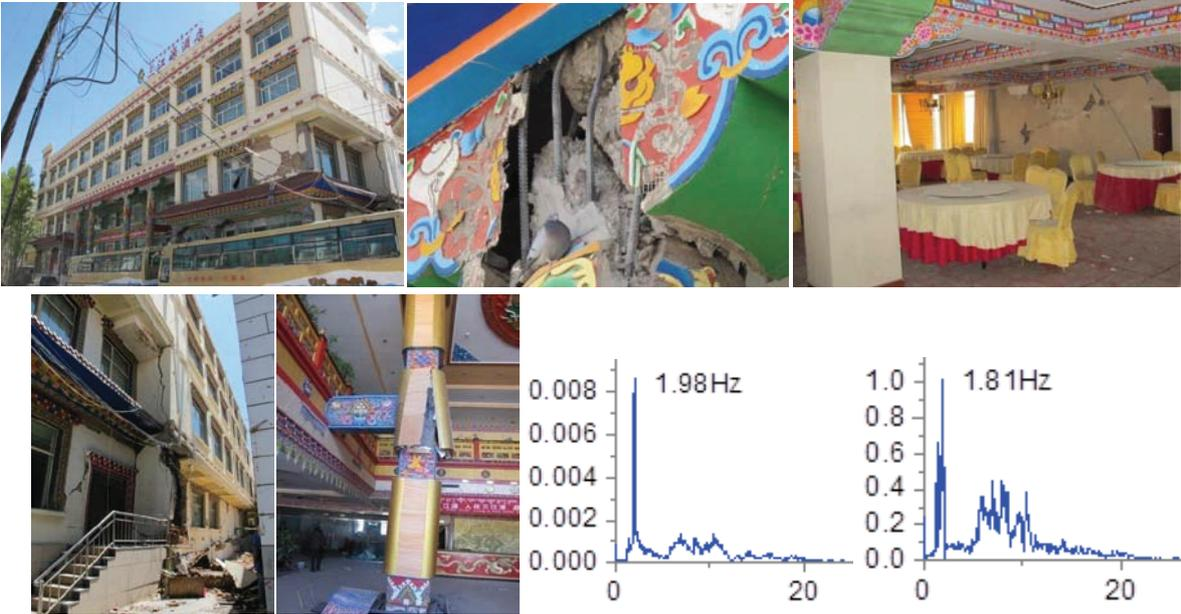
Figure 10. Damage of a 4-story RCF hotel building and its' NF (1.81Hz/1.98Hz) tested
