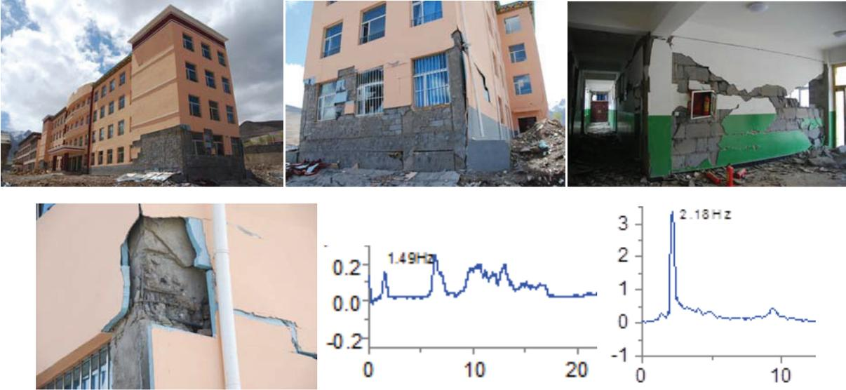
Figure 9. Damage of a 4-story RCF school building and its' NF (1.49Hz/2.18Hz) tested
