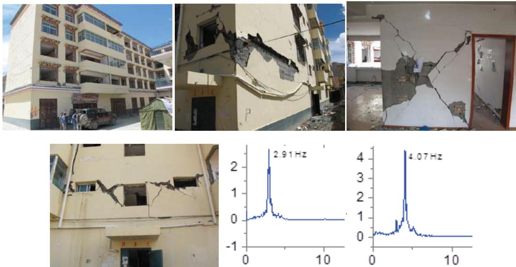
Figure 18. Damage of a 5-story BSWFSM residential building and its' NF (2.91Hz/4.07Hz) tested
