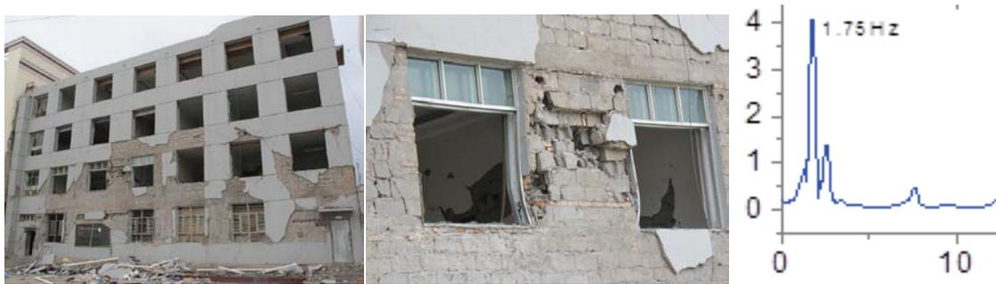
Figure 3. Seismic damage of a 4-story LCBCM office building and its' NF (1.75 Hz) tested
