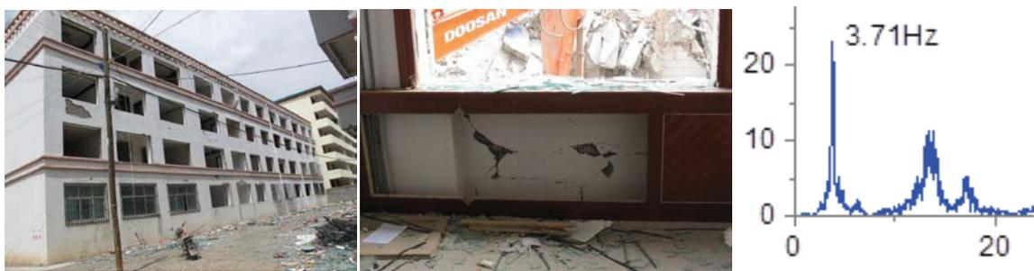
a) overview      b) damage of wall under window      c) NF tested (3.71Hz)
