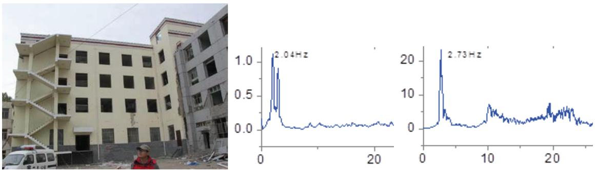
Figure 12. Damage of a 4-story RCF office building and its' NF (3.54Hz) tested
