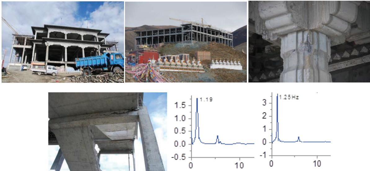
Figure 14. Damage of a 2-story RCF temple building and its' NF (1.19Hz/1.25Hz) tested
