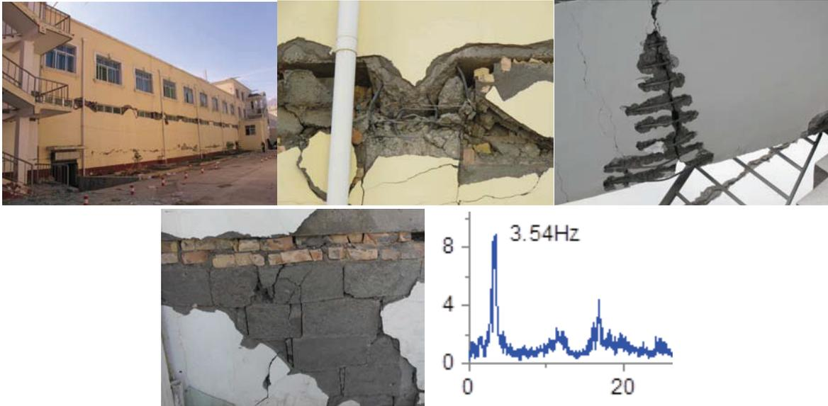
Figure 11. Damage of a 4-story RCF office building and its' NF (3.54Hz) tested
