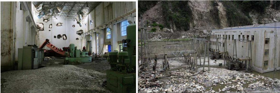
**Figure 6.** Damage of Shapai powerhouse due to rockfalls and flooding (left) and sediments from flooding due to penstock failure inundating the powerhouse and switchyard (right) (Wenchuan earthquake, China)
