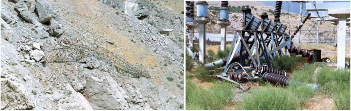
**Figure 5.** Failure of transmission tower caused by rockfall (left) and failure of switchyard components caused by ground shaking and settlement of fill material (right) (Sefid Rud dam; 1990 Manjil earthquake, Iran).
