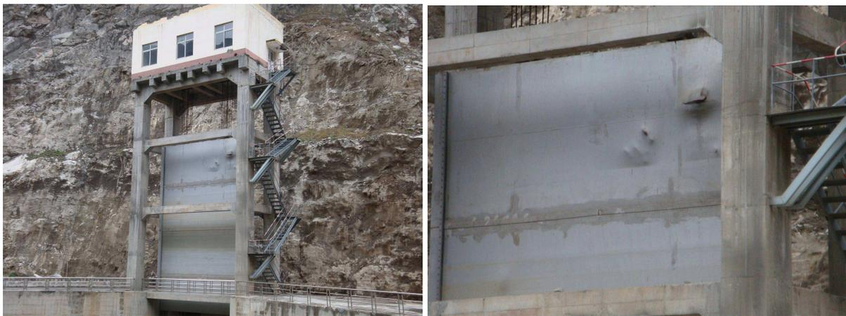
**Figure 3.** Damage of gate of power intake due to rockfall (Wenchuan earthquake, China)
