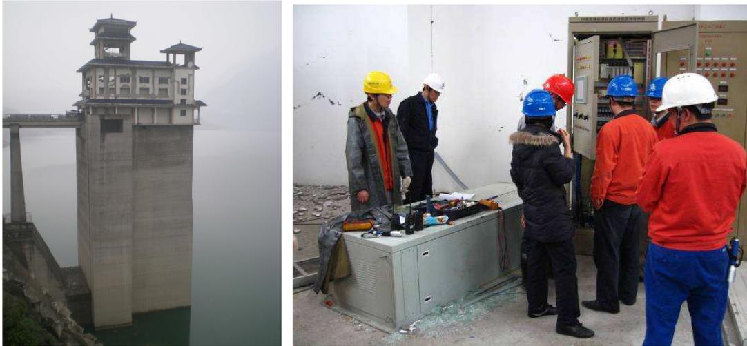
**Figure 2.** Intake tower and damaged gate room structure on top (left) and overturned control panel for operating the gates (right) (Zipingpu dam, Wenchuan earthquake, China)
