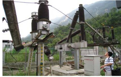
**Figure 3.2.** Most of transformers and circuit breakers are damaged in Beichuan 110kv Qimingxing substation
