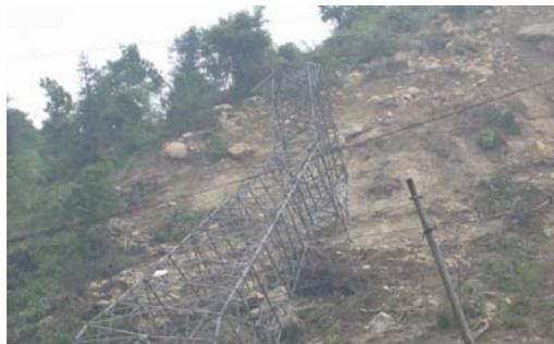
**Figure 3.5.** High voltage transmission tower toppled down and transmission line broken due to mountain landslide Yingxiu
