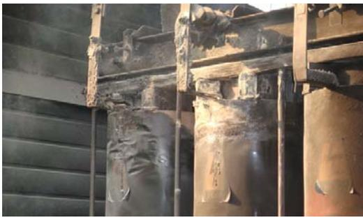
**Figure 3.3.** 10kv capacitor three-way reactor burnout and porcelain insulator burst in Guanghan Sanxingzhui substation
