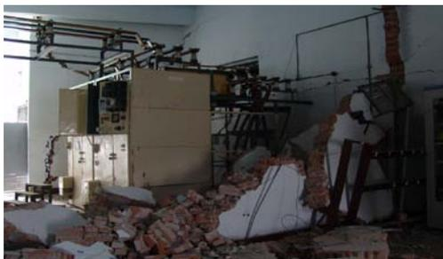
**Figure 3.7.** 6kv reserve high voltage switchgear smashed in Yuanmenba
