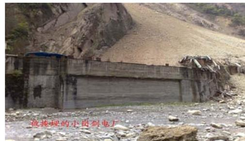
**Figure 3.8.** All equipments and buildings destroyed in Xiaogangjian substation
