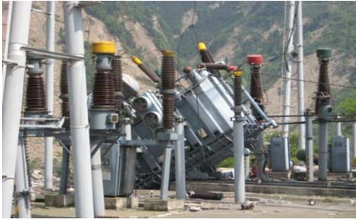
**Figure 3.1.** Transformer toppling down in 220kv Ertaishan substation
