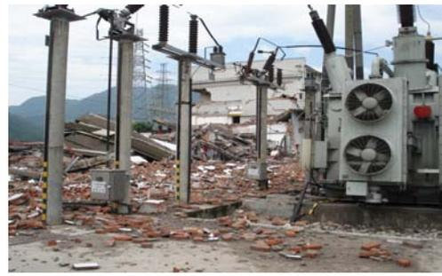
**Figure 3.4.** Main control room collapsed, transformer displaced and oil leaked
