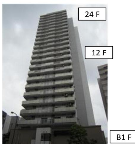
**Figure 2.** Photograph of building D and locations of accelerographs.
