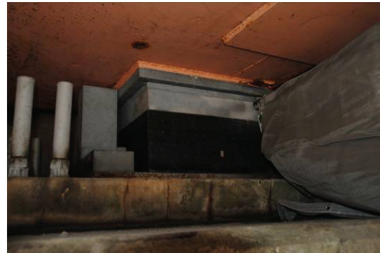
(b) An elastomeric bearing which did not suffer damage during 2011 great east Japan earthquake
