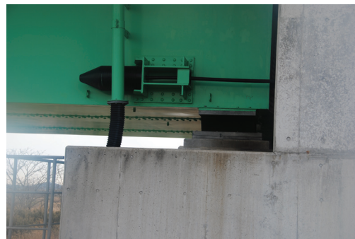
(b) Elastomeric bearing and cable restrainer without damage
