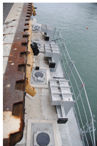
(b) Steel bearings and stoppers on P10
