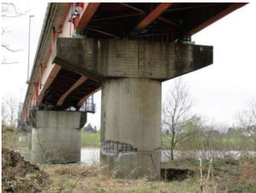
Photo 1. Shear failure due to insufficient termination of longitudinal bars at cut-offs (Fuji Bridge, courtesy of Hoshikuma, J., PWRI)
