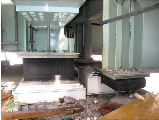
(a) Offset of left girder by 0.5m due to rupture of elastomeric bearings (NEXCO East)
