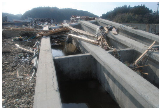
Photo 10. Overturned Span S8
