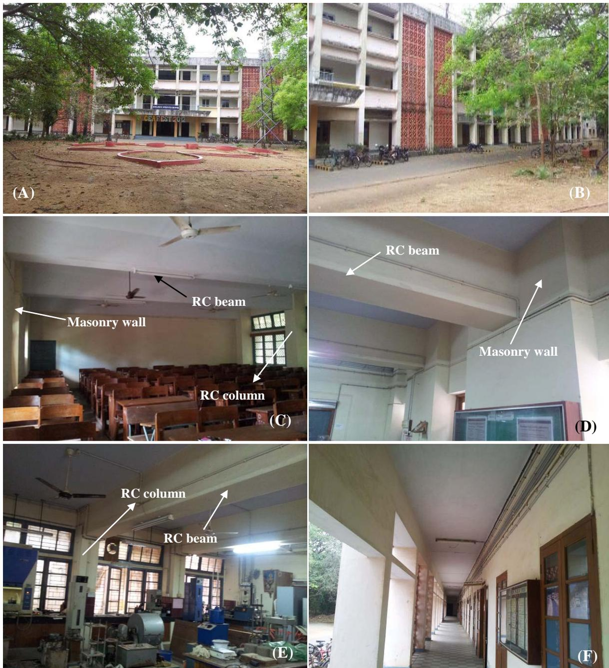
**Figure 4.** (A-B) Exterior views, (C-D-E) RC beam supported on masonry wall and RC column, F: Corridor
