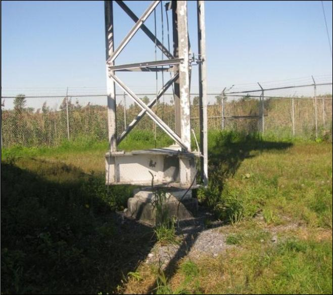
b) Mast pinned-base connection
