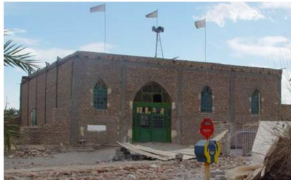
**Figure 1.** A confined masonry building that did not collapse after the Bam earthquake, Iran, 2003
