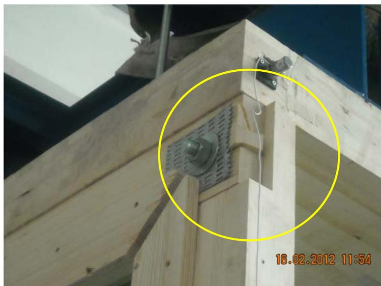
**Figure 9.** Detail of damage in the wooden frame
