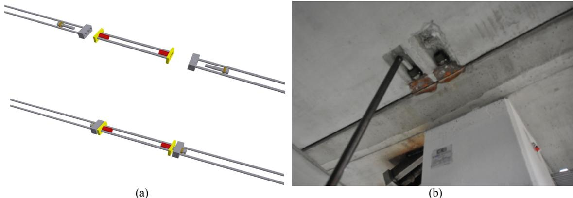
**Figure 4.** (a) Loosen and activated connection system in its bare configuration. (b) Activation of the loosen bolts to provide continuity to the longitudinal bars crossing the beam-column joint.
