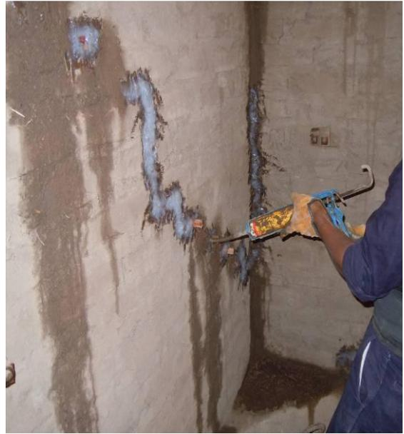
Injecting mud-based grout
