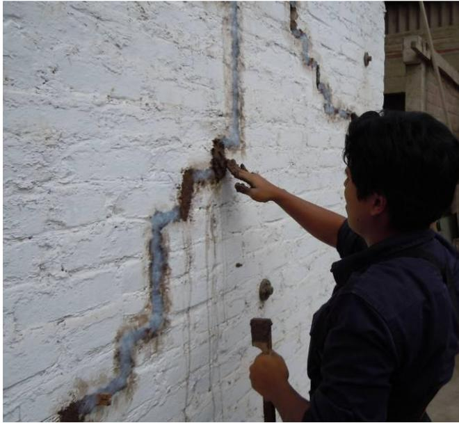
Filling thicker cracks manually
